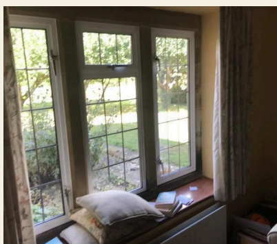
PRE-WORKS SURVEY · PROJECT RECORD
