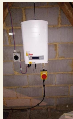
PRE-WORKS SURVEY · PROJECT RECORD
