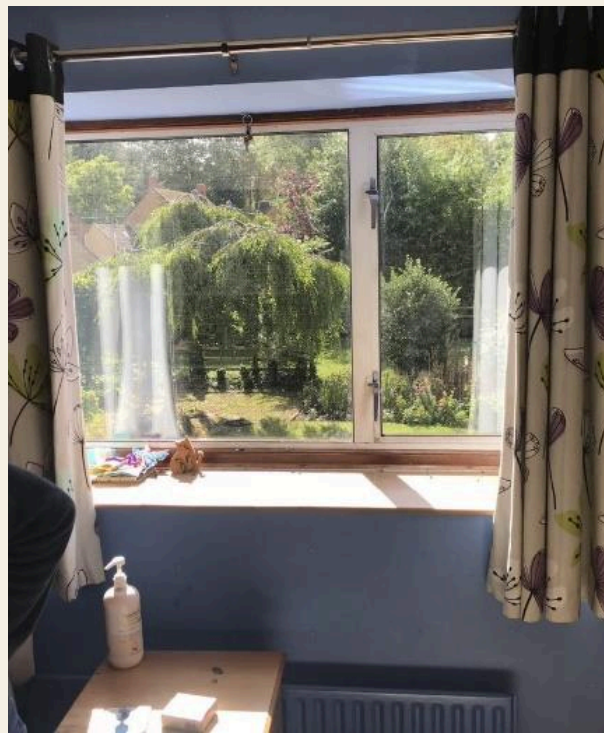
PRE-WORKS SURVEY · PROJECT RECORD
