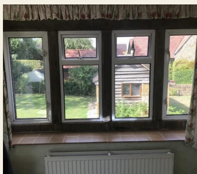
PRE-WORKS SURVEY · PROJECT RECORD
