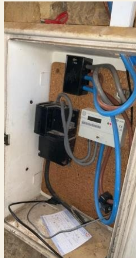
PRE-WORKS SURVEY · PROJECT RECORD
