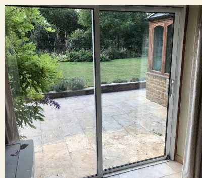
PRE-WORKS SURVEY · PROJECT RECORD
