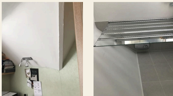
PRE-WORKS SURVEY · PROJECT RECORD
